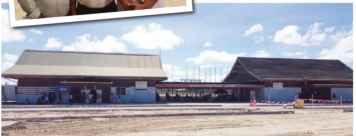
Upgrade works at Tarawa International Airport have begun.
